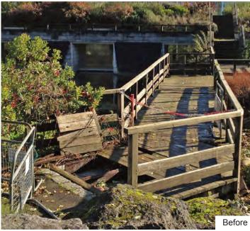
We can provide expert solutions for all types of footbridge or raised walkways, including removal and planning for sensitive and public facing projects. This 18 metre timber constructed pedestrian bridge at Kew Gardens was surveyed, re-planned, removed and re-built in just 3 weeks.
